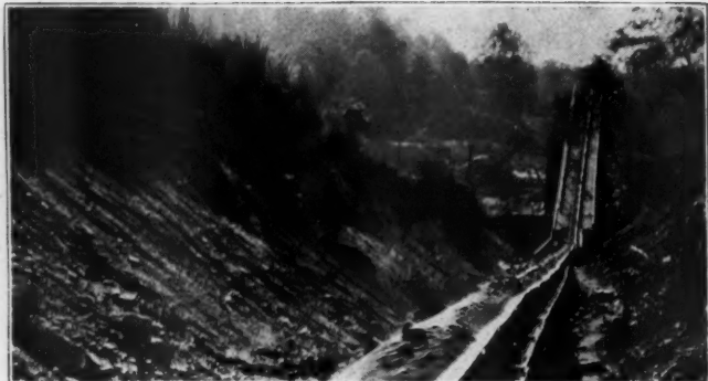
Conveyor from Grizzly to top of incline. Little Falls
